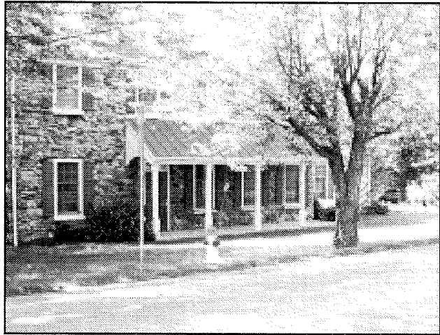
New construction in Lederach that illustrates these building design standards
